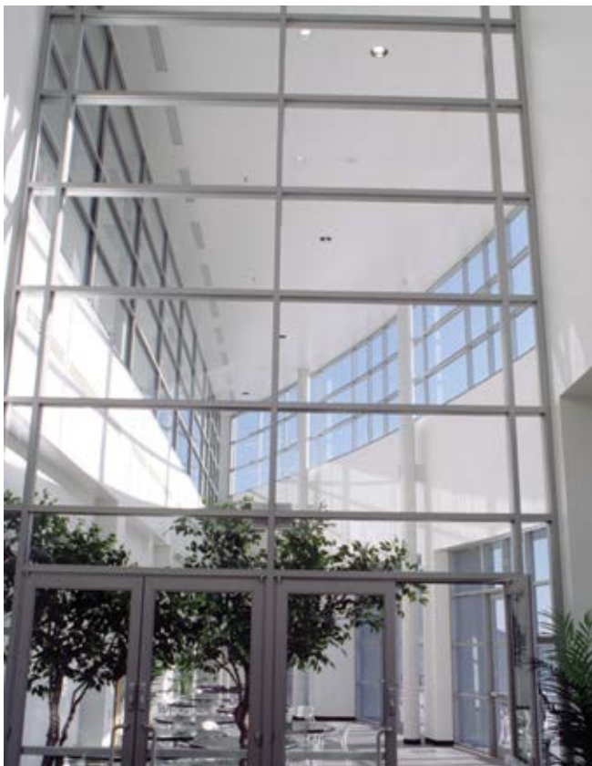
Credit: Warren Gretz / NREL
