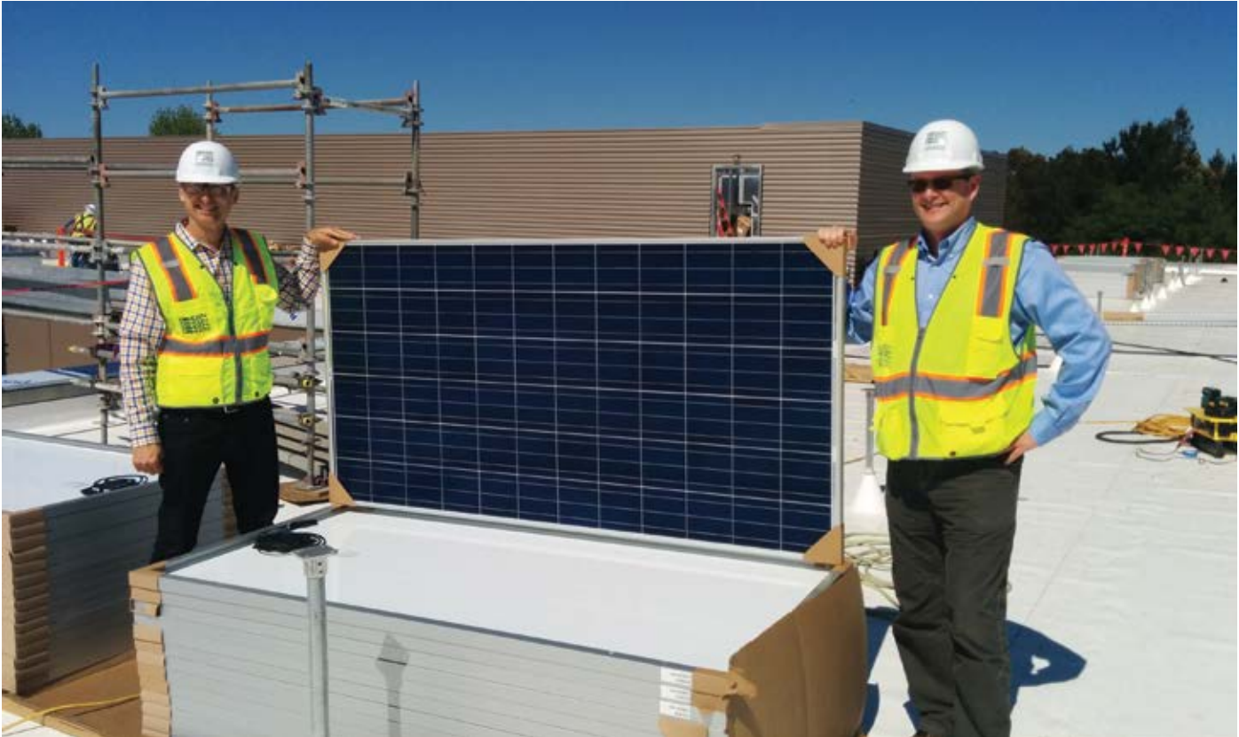
Peter Rumsey and the developer Jim Gaither Jr. on the roof of the 1400 Page Mill Road Net Zero Energy Building.
