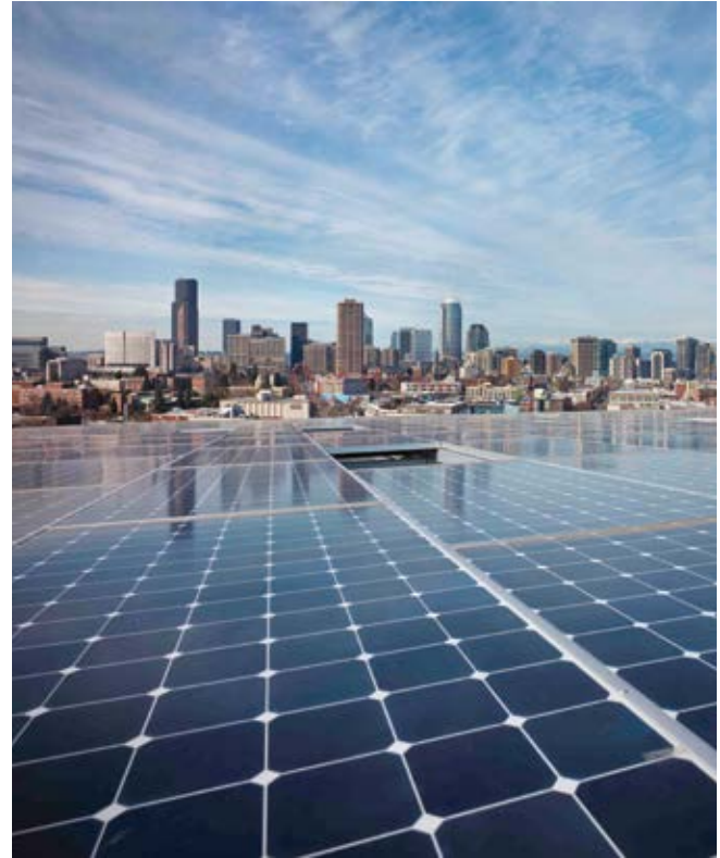
Rooftop of the Bullitt Center, one of the nation’s largest solar powered net zero energy commercial office buildings, in sunny Seattle. Credit: Benjamin Benschneider
