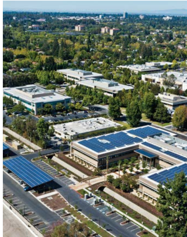
Credit: Steve Proehl Sun Light & Power
