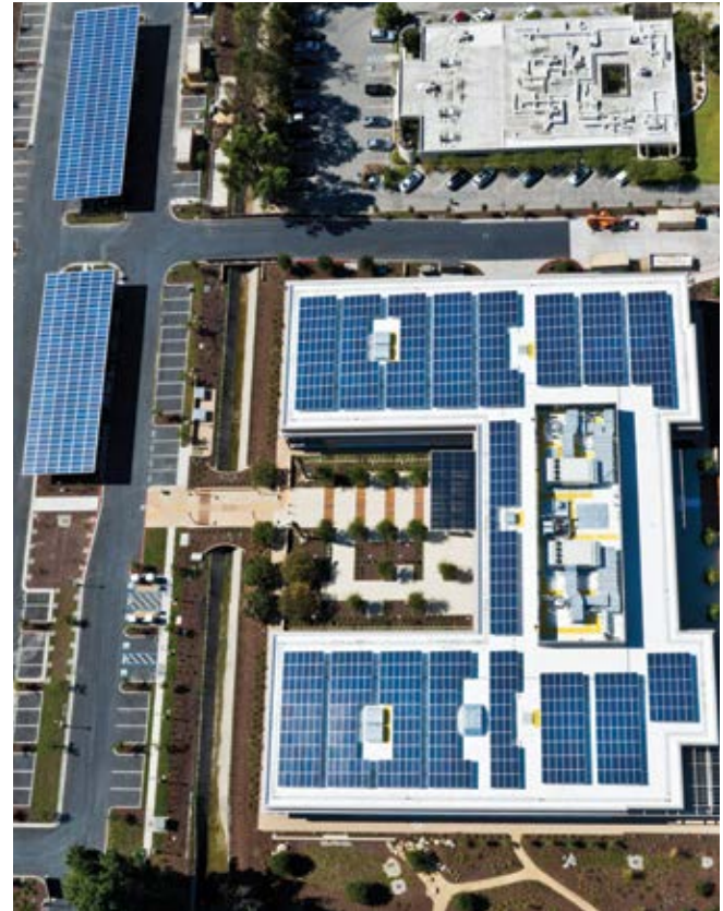
Credit: Steve Proehl Sun Light & Power
