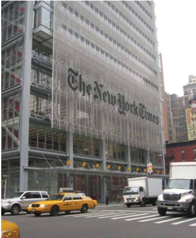
The 52-story New York Times building used efficiency measures to reduce electricity use by 24% and heating and cooling by over 50%. Credit: Virginia Cahill
